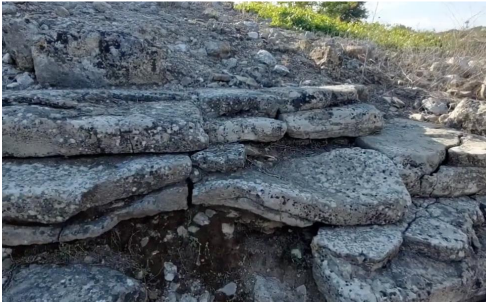
Fig. 7. Aspendos, Turkey. This screenshot shows how a stone slab experienced plastic deformation due to an unknown mechanism ( https://www.youtube.com/watch?v=ocVplh2dvqM ).
